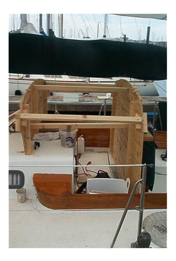
Using 3 pieces ¼" of "Bendy Ply". This is a special plywood with all the grain running in one direction. You can bend this ply 180. Laid on top of the form, epoxied together will form a stiff structure. Let cure overnight before removing the clamps
